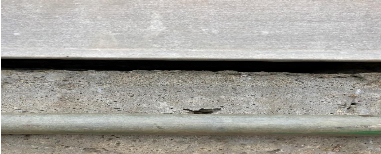
Unsealed gap between Roof and Concrete walls
