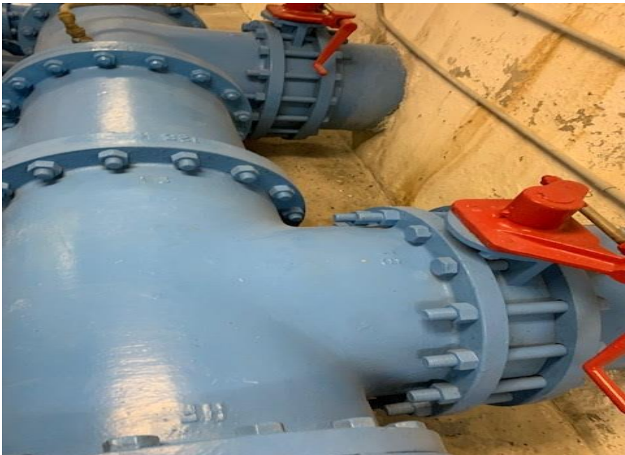
Piping manifold with the two-intake piping on the outside of the reservoir
