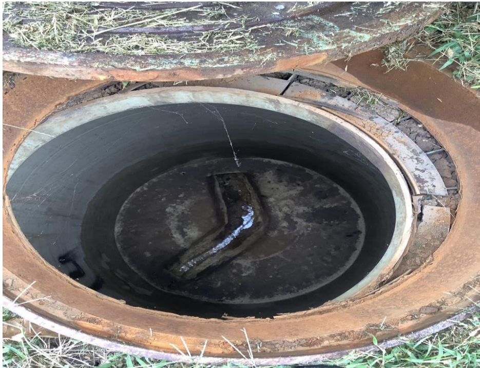
Manhole with a Bad Ring & Riser missalined
