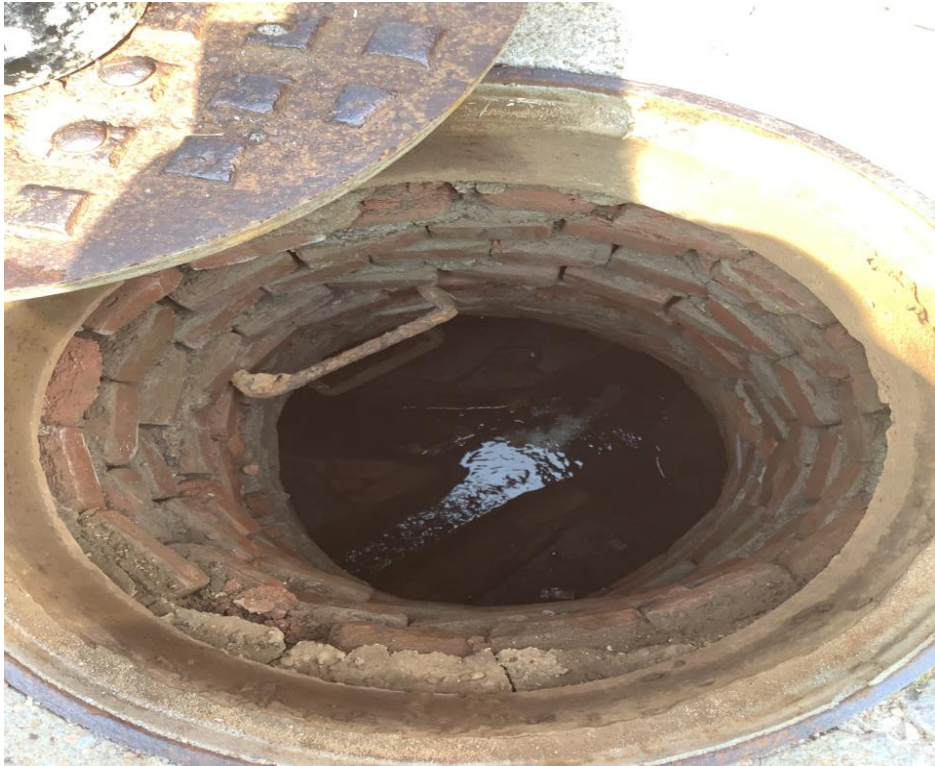
Manhole that needs lined
