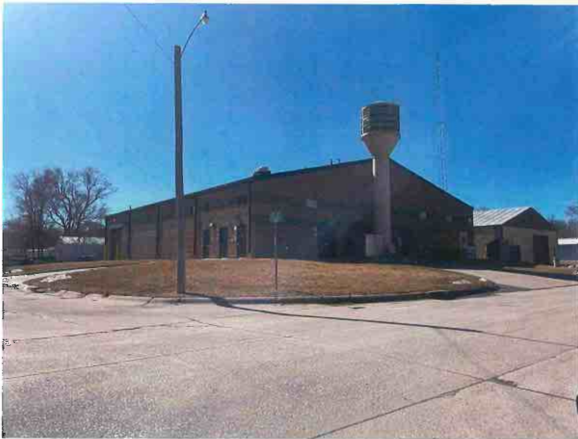
Figure 2 Auburn Water Treatment Plant
